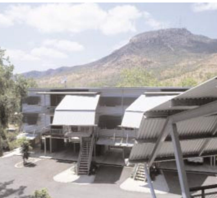
LEFT: BUILDINGS SUCH AS THE LAVARACK ARMY BARRACKS IN TOWNSVILLE HIGHLIGHT THE ENVIRONMENTAL CREDENTIALS OF STEEL
